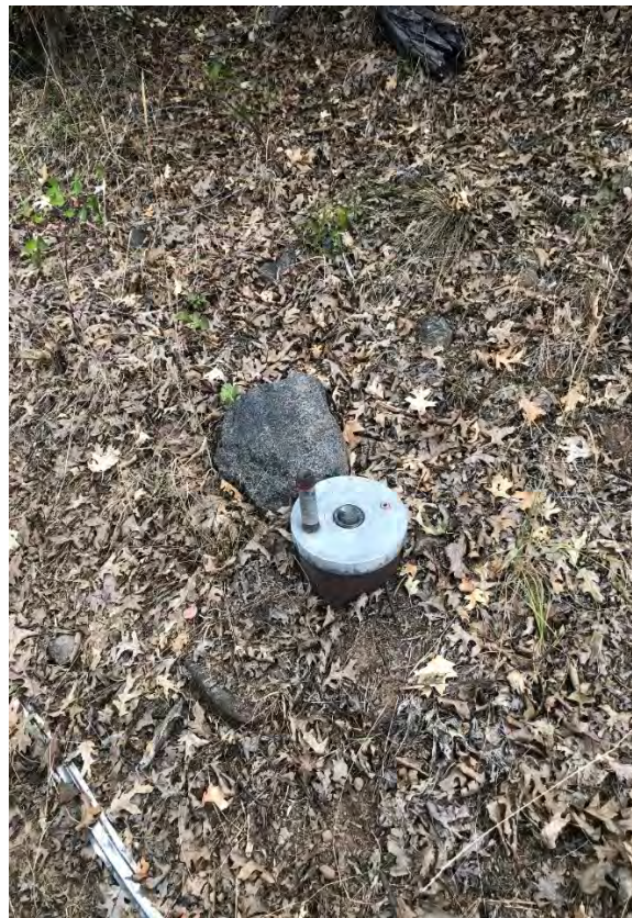
8 inch capped well
